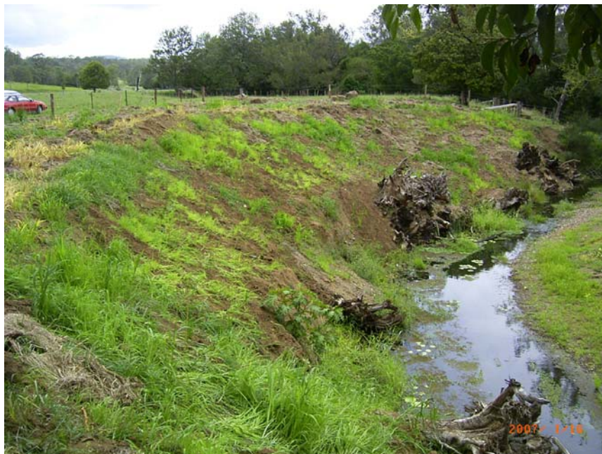
Cork Site – Looking downstream at engineered log jams 1, 2 & 3 and revetment logs.
