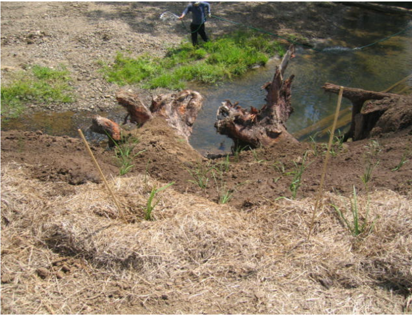
Garmany Site – Engineered log jam number 2 from top of bank (note tree planting on upper bank and Iomandra longifolia planted on steeper bank)
