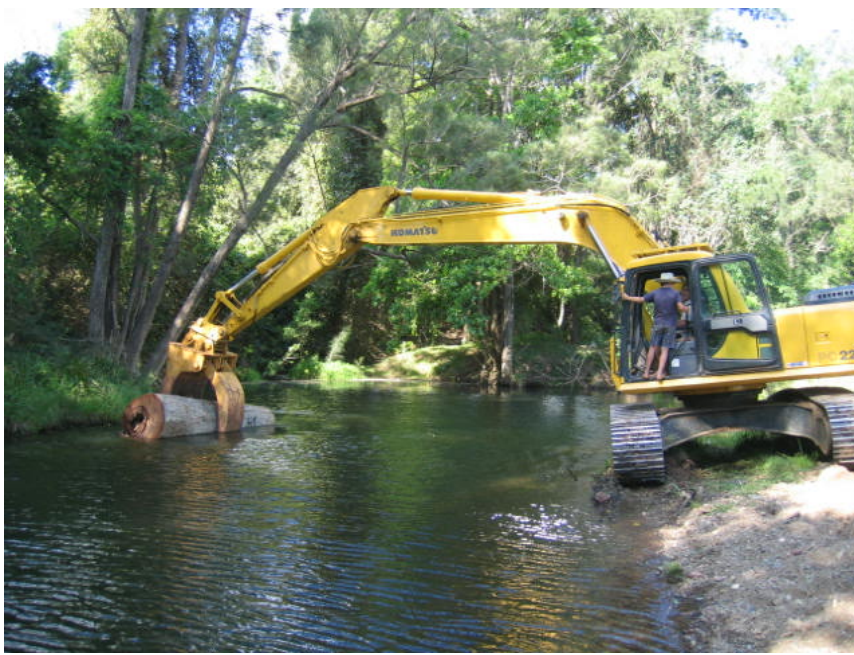
Cork Site – Hollow habitat log placement in pool upstream of eroded bank
