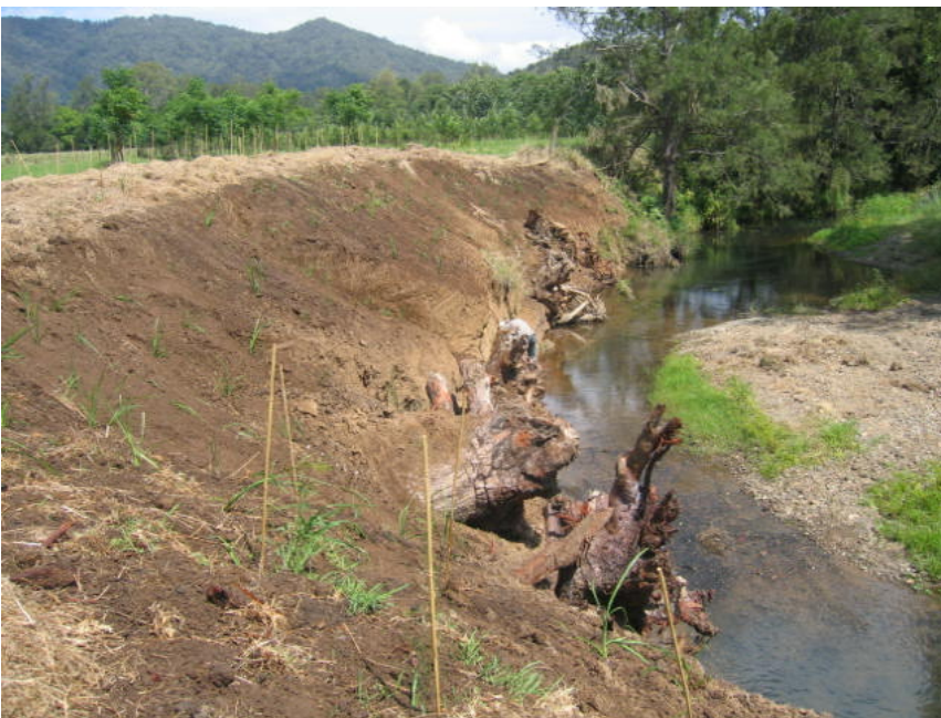
Garmany Site – Looking downstream at engineered log jams 1, 2 & 3 and revetment logs.
