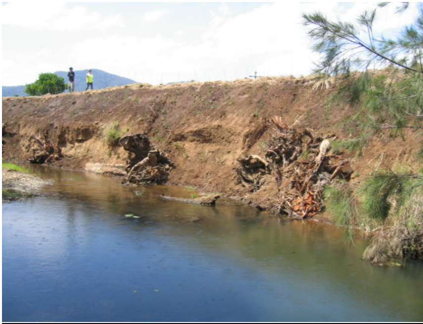
Garmany Site – Looking upstream at engineered log jams 1, 2 & 3 and revetment logs.
