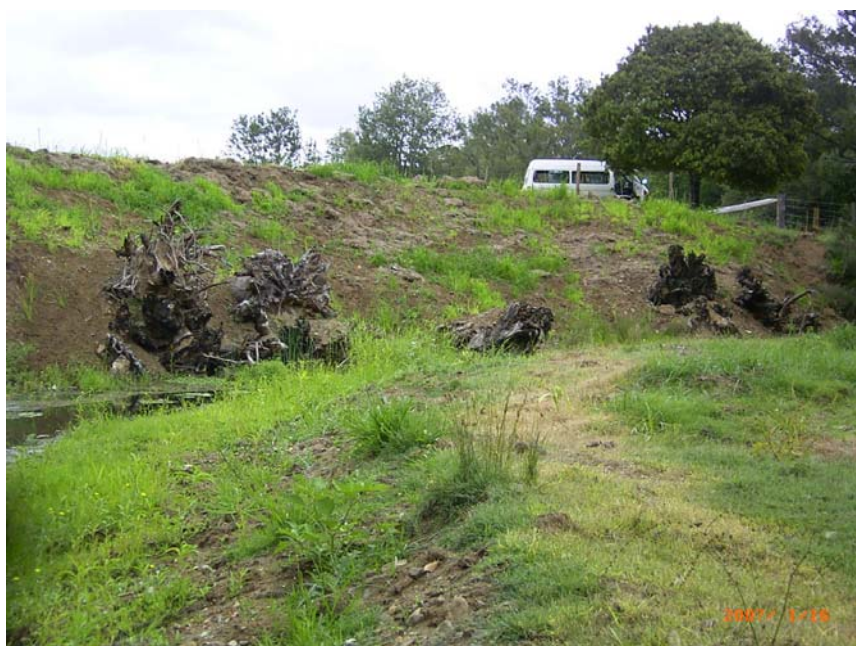
Garmany Site – Looking downstream at engineered log jams 1, 2 & 3 and revetment logs.
