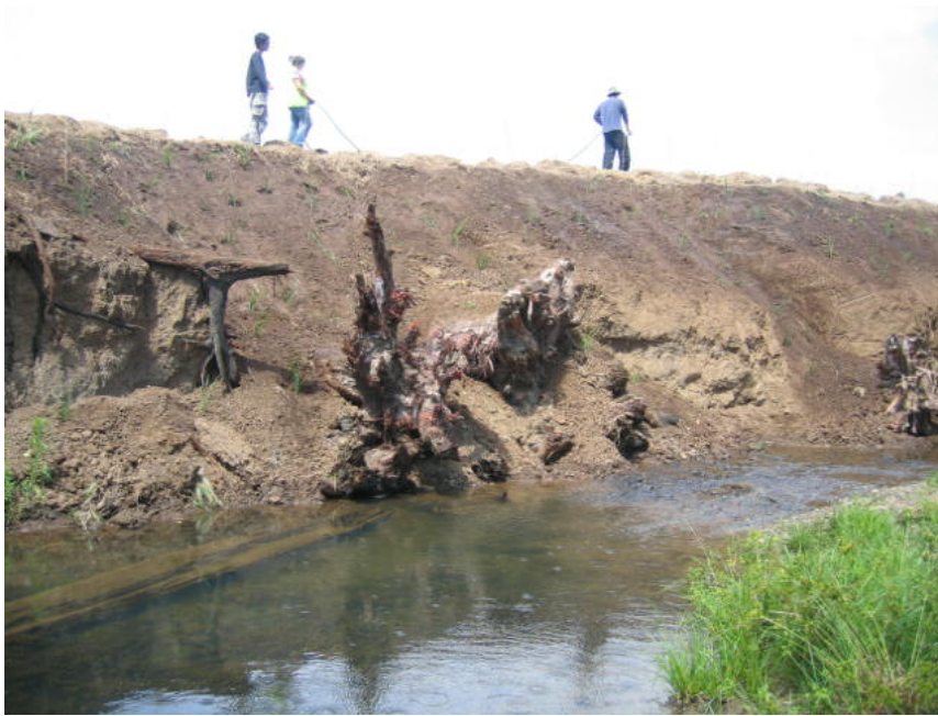
Garmany Site – Looking downstream at engineered log jams
