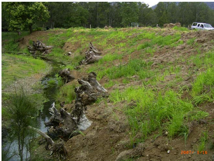
Cork Site – Looking upstream at engineered log jams 1, 2 & 3 and revetment logs.
