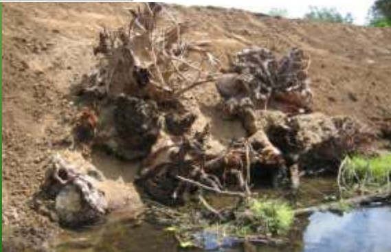
Hannu Creek Wood Reintroduction - Engineered Log Jam (ELJ) Configuration
