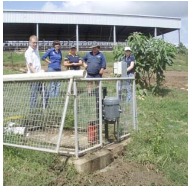
Property owners Greg and Michelle Anderson view their new automated effluent sludge pump with BMRG and QDO representatives.
