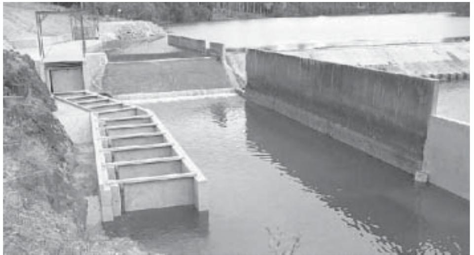
*Upgraded fishway on the Mary River Barrage, and three barramundi that successfully negotiated the new fishway*
