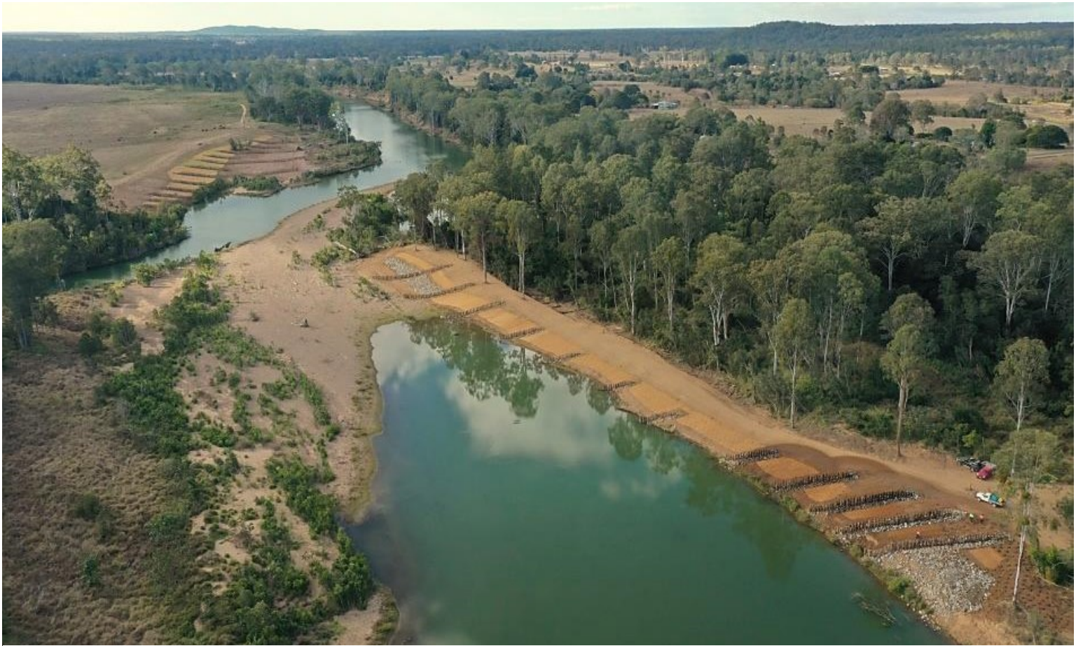
After bank stabilisation works at Tiaro, September 2023
