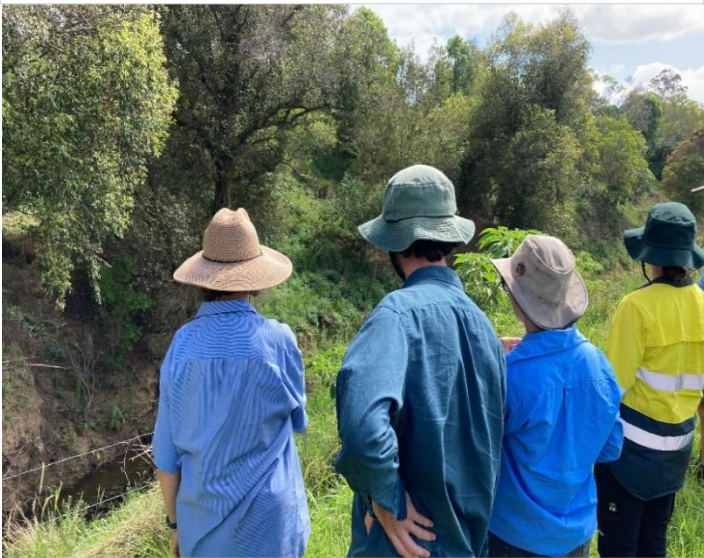
Landholder, Kerry Murray with, Kyle (Noosa District Landcare), Alana (MRCCC) and Nicole (Noosa District Landcare) inspecting the condition of the creek bank after flooding at the Murray's Mary River Property
