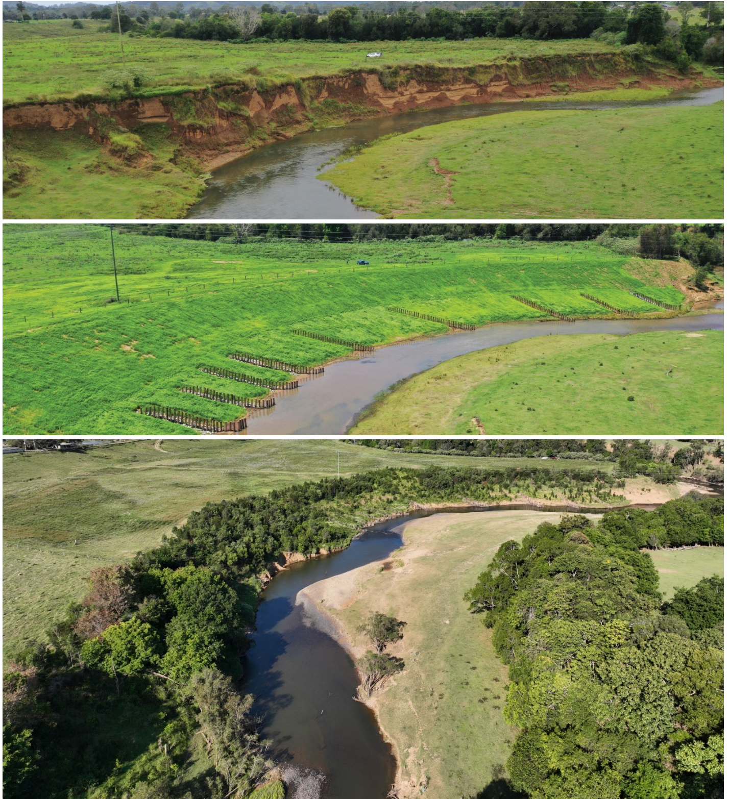
Mary Valley large scale riverbank remediation. Top photo, March 2021, middle October 2021, below October 2025.
