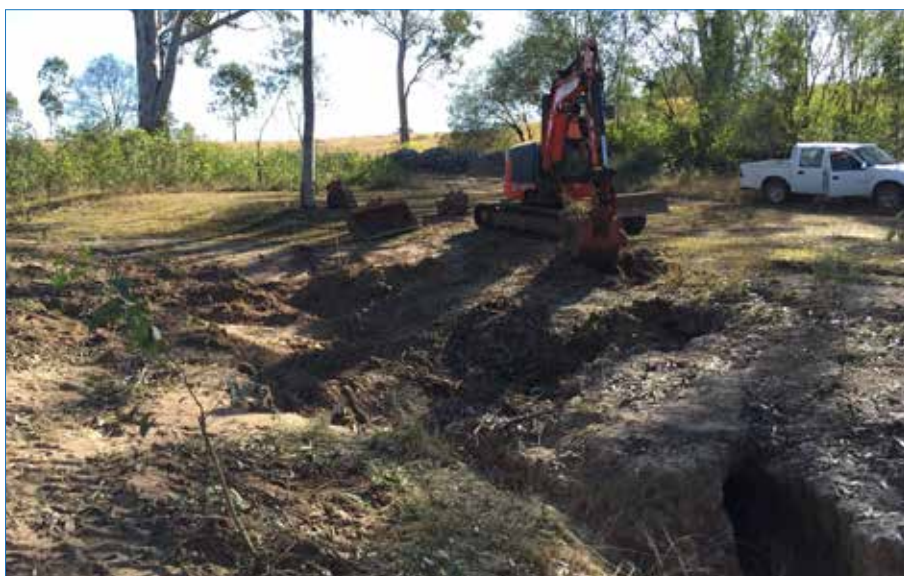
Photo 36 Another tunnel before it was collapsed.
