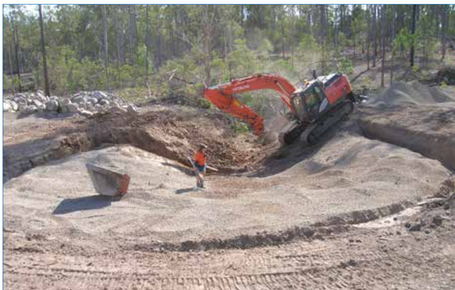
Photo 23 Excavation of bottom cut-off trench and gravel placed on chute batter.
