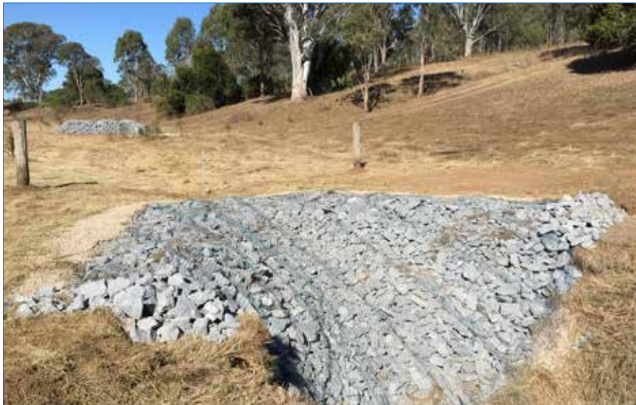
Photo 15 Completed chute with stock exclusion fencing in place – looking upstream.
