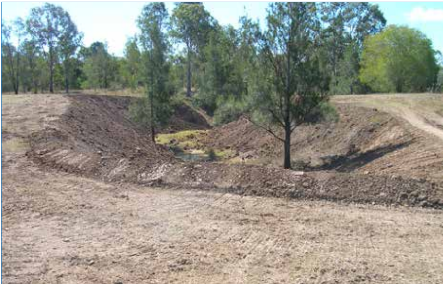
Photo 114 Completed: looking down the old by-wash.
