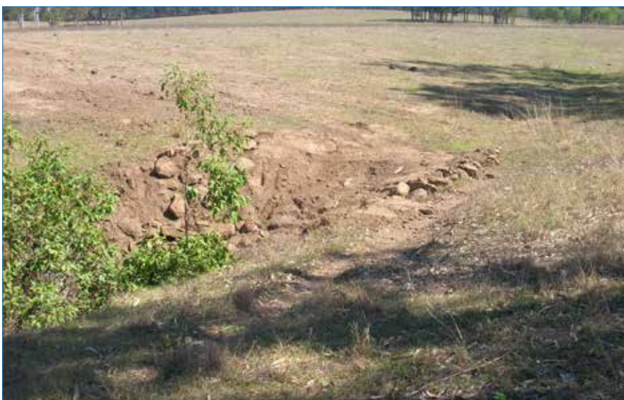
Photo 109 Small gully on the end of the by-wash stabilised with rock-fill chute (using locally sourced larger rock and gravel).
