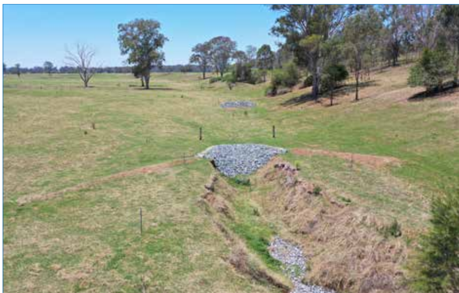
Photo 17 Three months post-construction. October 2020 at the beginning of first wet season.
