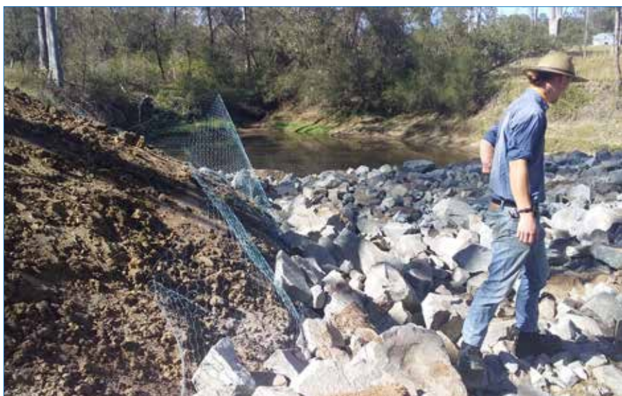
Photo 94 Netting placed along the batter before adding rock to hold it in place.
