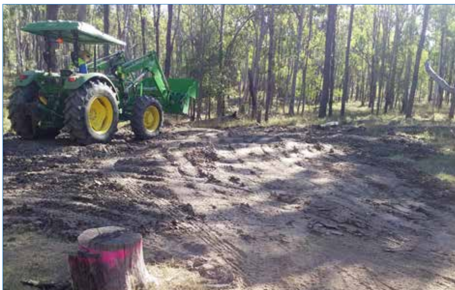
Photo 55 Filled gully head.
