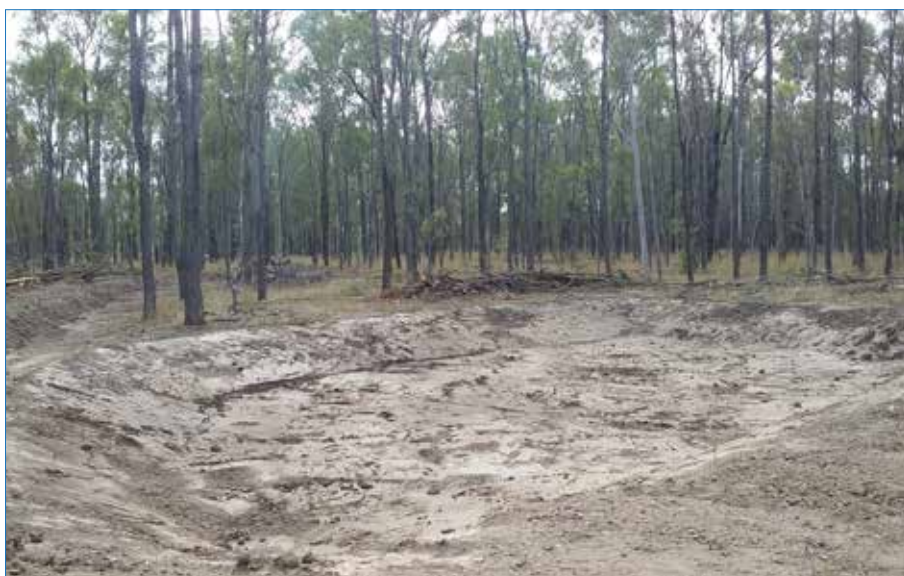
Photo 51 Detention dam, complete with by-wash, surveyed along ridge line.
