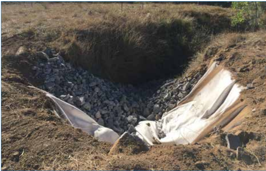
Photo 127 Drop structure completed – looking downstream.
