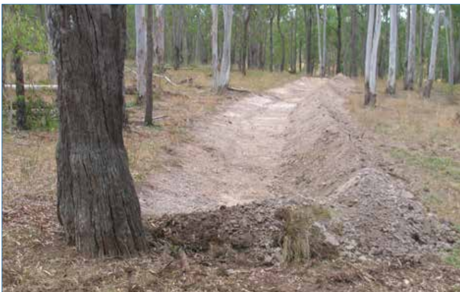
Photo 60 Short top diversion bank above the start of the main diversion bank.
