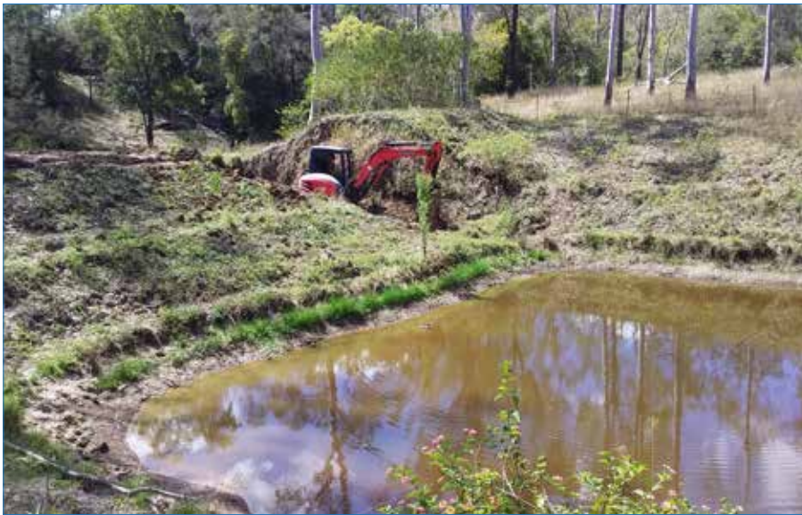
Photo 89 Excavation of crest.
