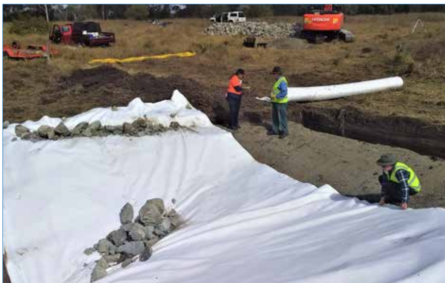
Photo 73 Geofabric placed to cover entire structure.
