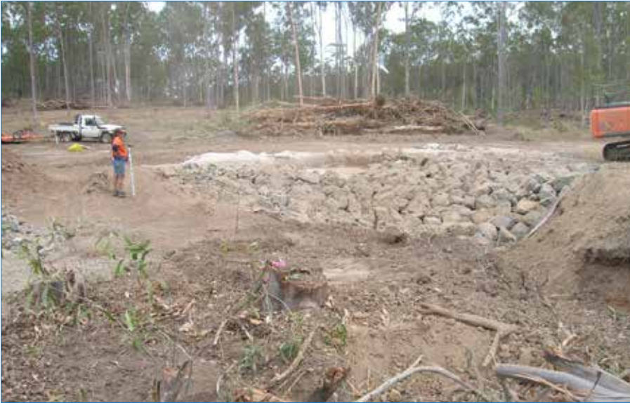
Photo 26 Rock-fill on the chute close to finished.
