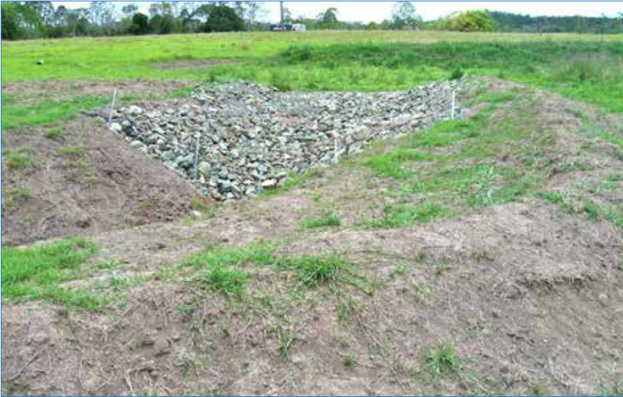
Photo 82 Rock chute and dam wall looking upstream after rain. Ground cover is starting to establish.
