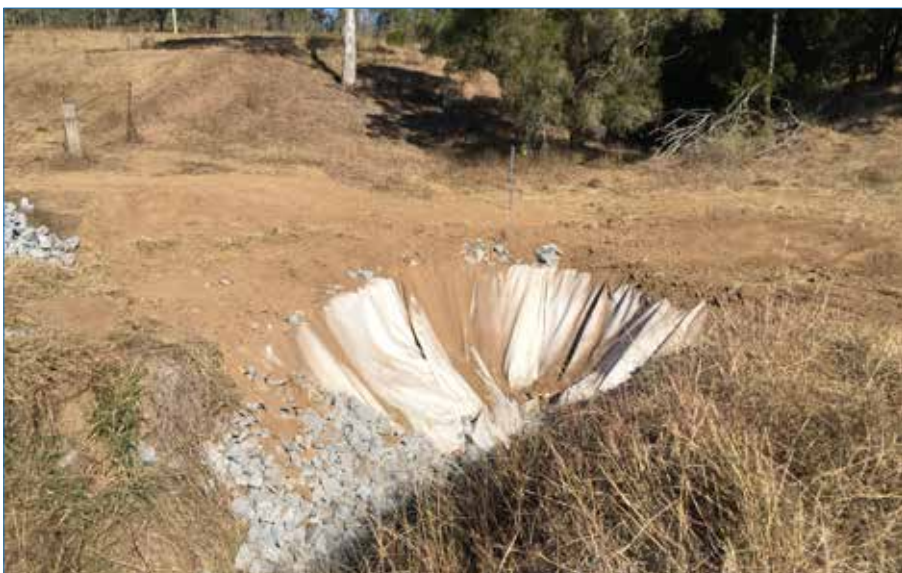
Photo 126 Drop structure completed – looking upstream.
