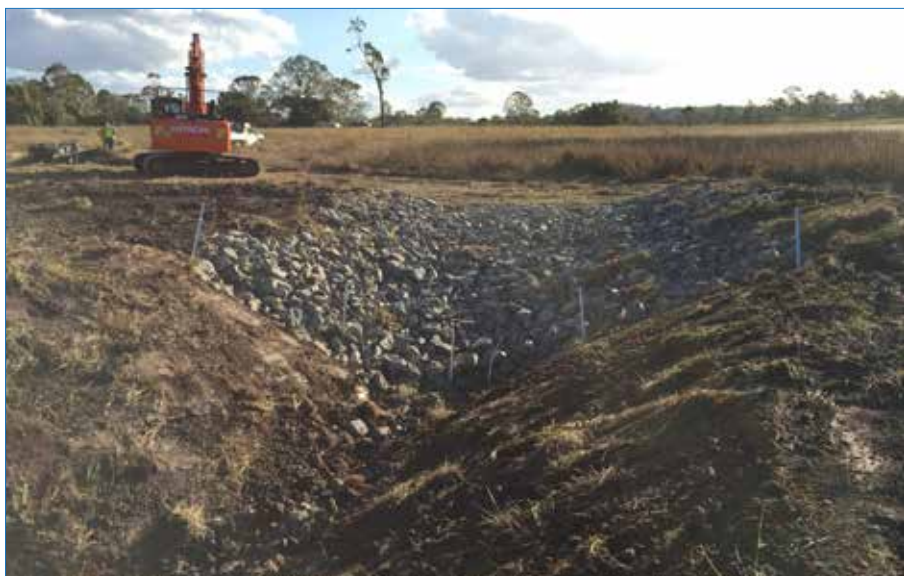
Photo 79 Rock chute complete July 2020.
