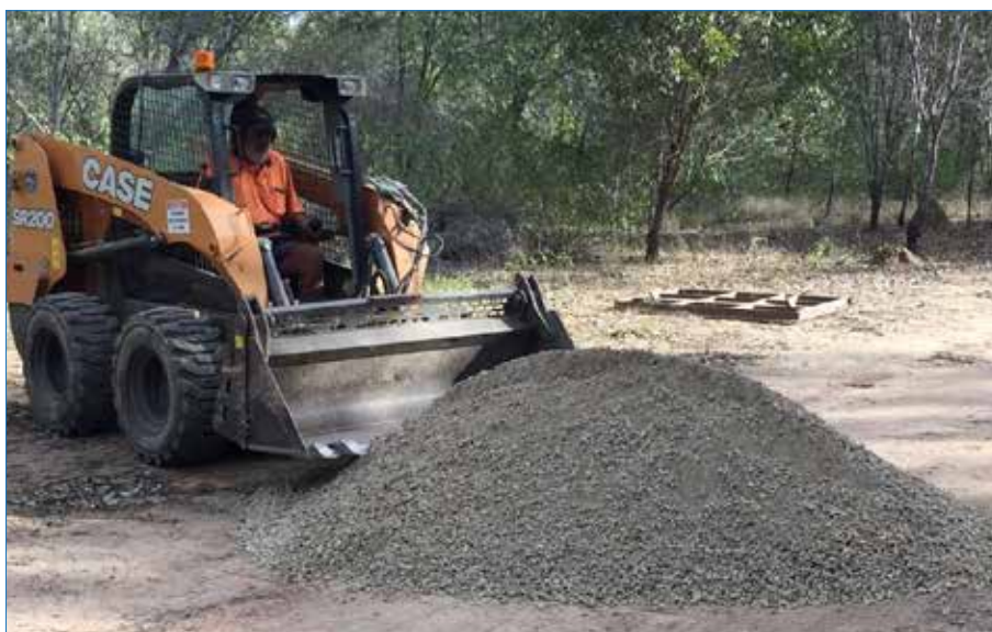
Photo 42 Gravel road base dumped in position on the driveway ready to be shaped into a whoa boy.
