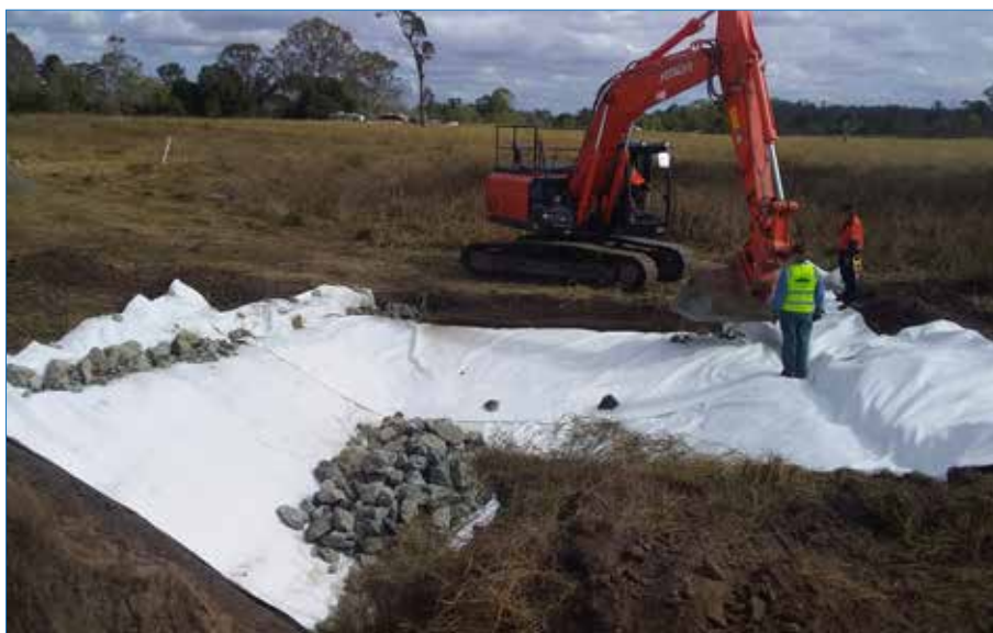
Photo 74 Geofabric completed and rock goes on.
