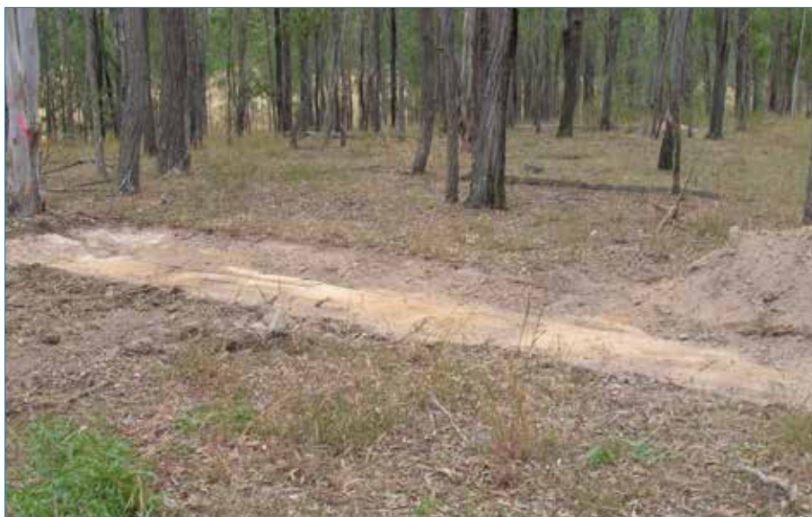
Photo 61 Short top diversion bank level sill outlet showing the grassed slope where water spreads.
