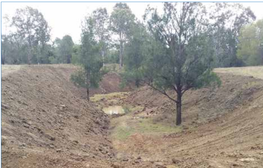
Photo 108 By-wash gully walls battered and topsoiled.
