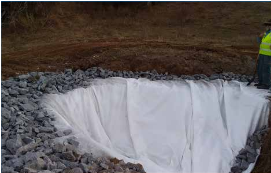
Photo 124 Top and bottom cut-off trenches and side wall trenches filled with rock.
