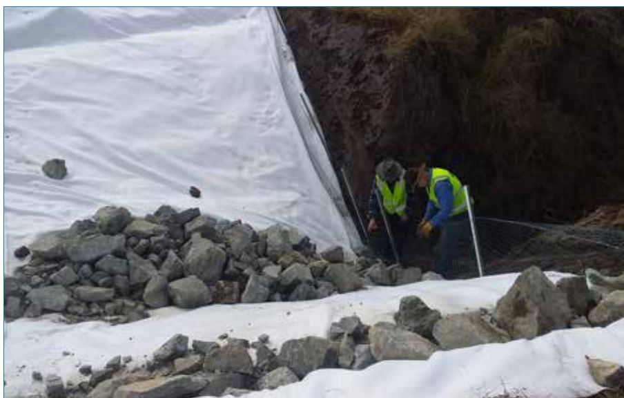
Photo 75 Netting fence constructed in bottom cut-off trench.
