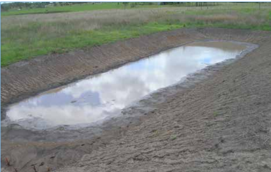
Photo 84 Detention dam after first rain event.
