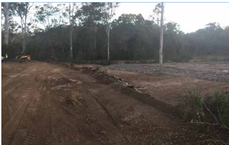
Photo 41 Log and gravel line along roadside to divert water away from the completed structure.
