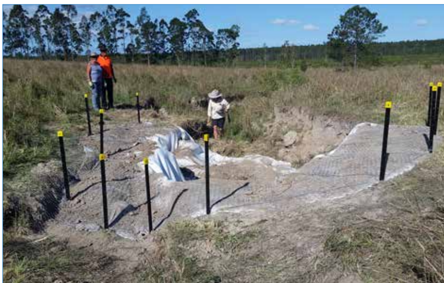
Photo 134 Tension wire around the crest.
