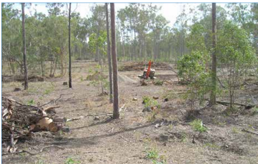
Photo 30 Survey line for wing wall.
