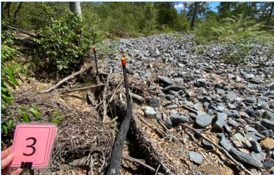
Photo 44 Ongoing maintenance of silt trap weirs below rock mattress.
