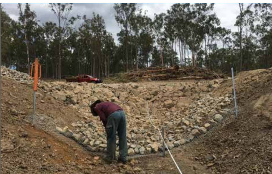
Photo 28 Completed rock chute. Fence constructed at the bottom end of the structure to stop rocks rolling away during rainfall events.
