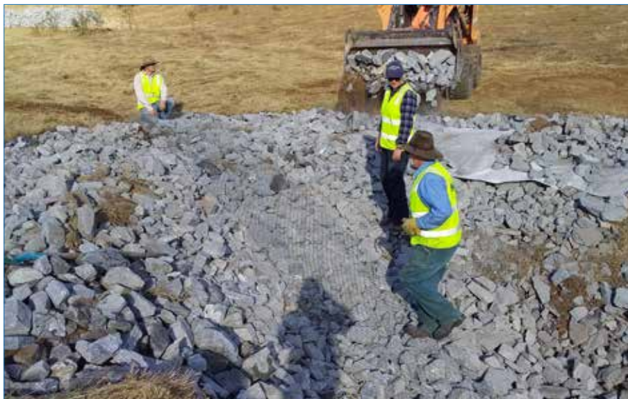
Photo 11 Lengths of wire netting placed over the rock chute and attached to netting in cut-off trenches.
