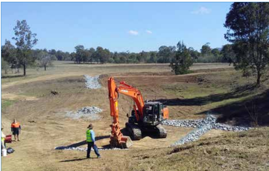
Photo 113 Completed: from the top rock chute captures water from overland flow.
