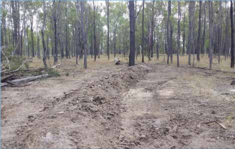
Photo 52 Detention dam by-wash surveyed almost level, with log lines in place.
