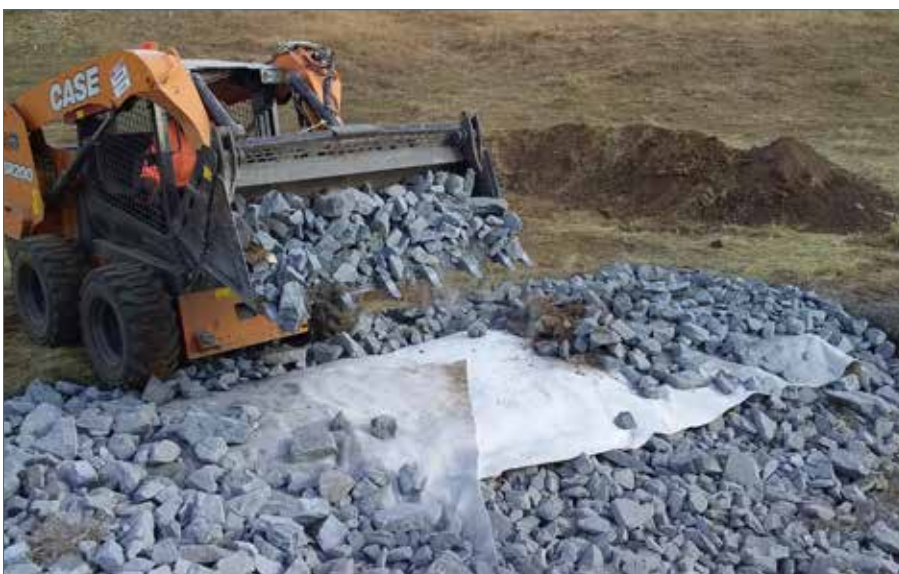
Photo 10 Gravel and rock placed over the fabric.
