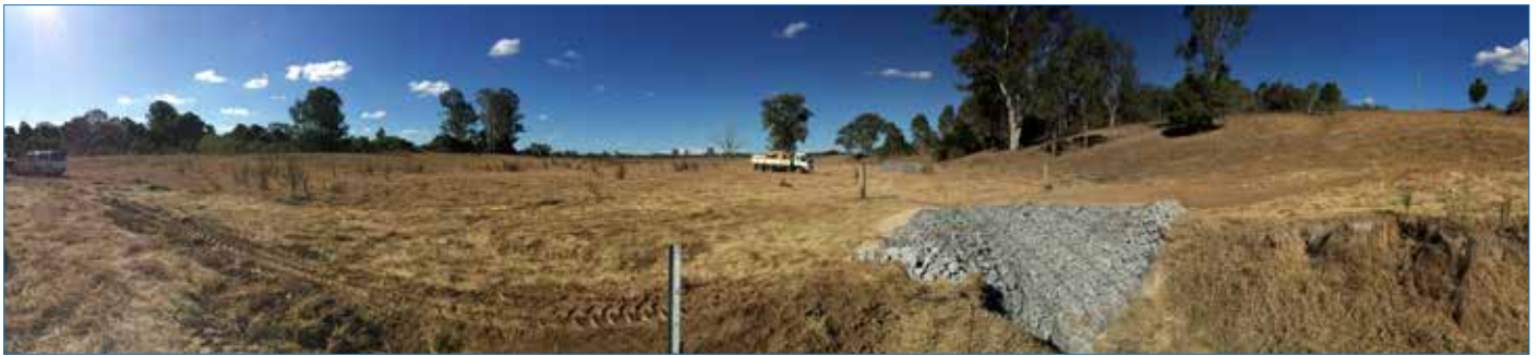
Photo 14 Soil from excavation used for diversion wing bank construction.
