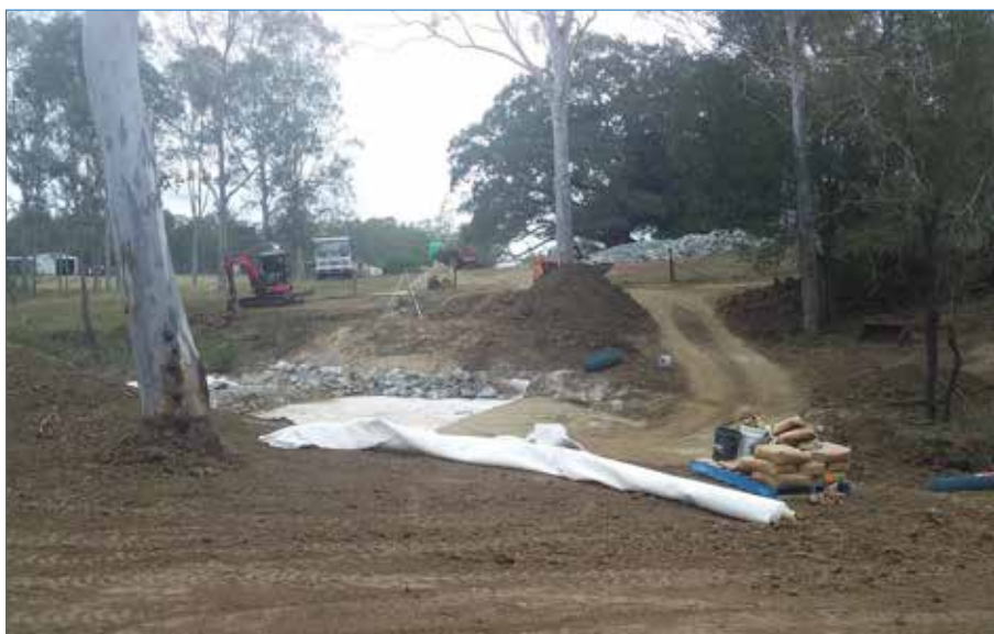
Photo 93 Placement of materials.
