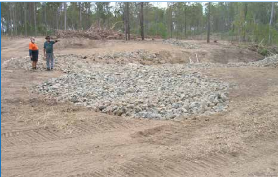
Photo 27 The depressions in the gully above the crest were filled with small rock and compacted.
