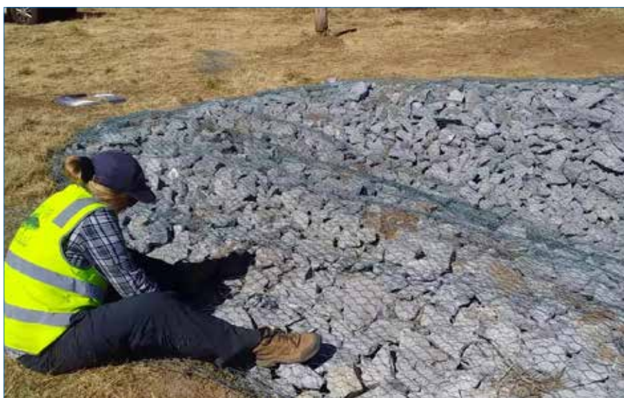
Photo 12 Wire netting laced together with 2.5 mm plain wire, to form one single large gabion.
