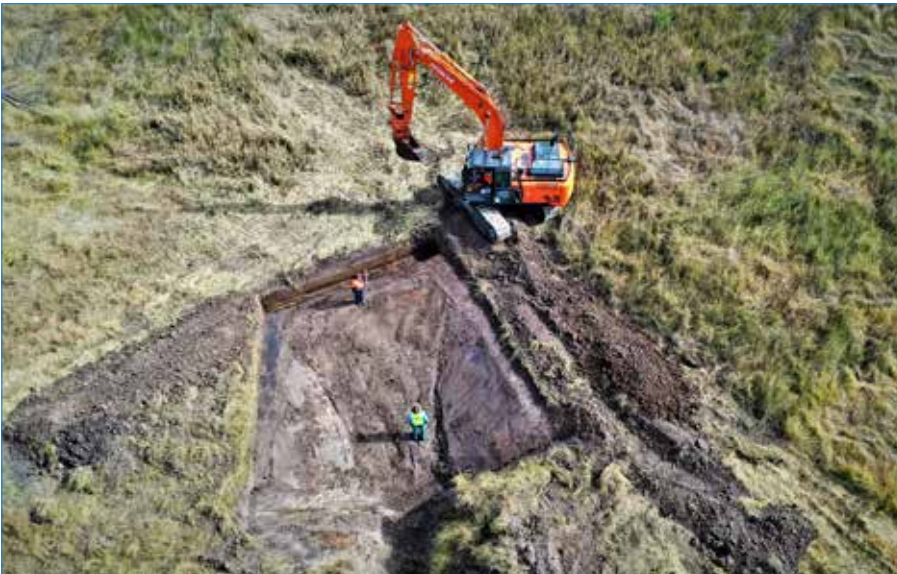
Photo 71 Gully head chute shaping completed.
