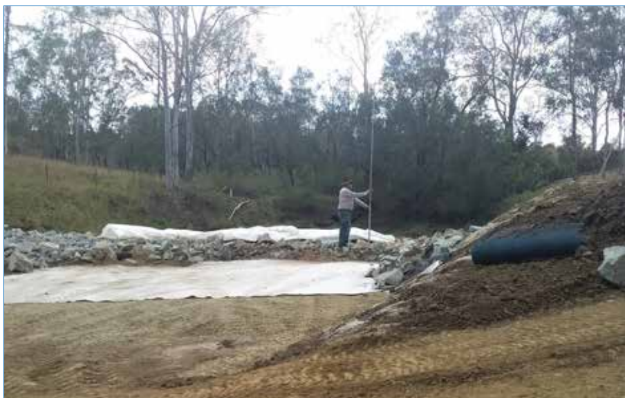
Photo 92 Layering – first bentonite, gravel, Texcel 400R fabric then rock. Continuous surveying to ensure rock mattress was level across the width.
