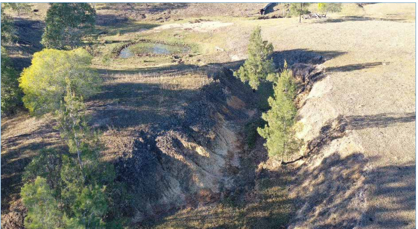
Photo 103 Looking upstream along the eroded by-wash.
