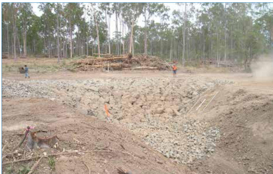
Photo 29 Some excess rock placed downstream of the apron and the fence.
