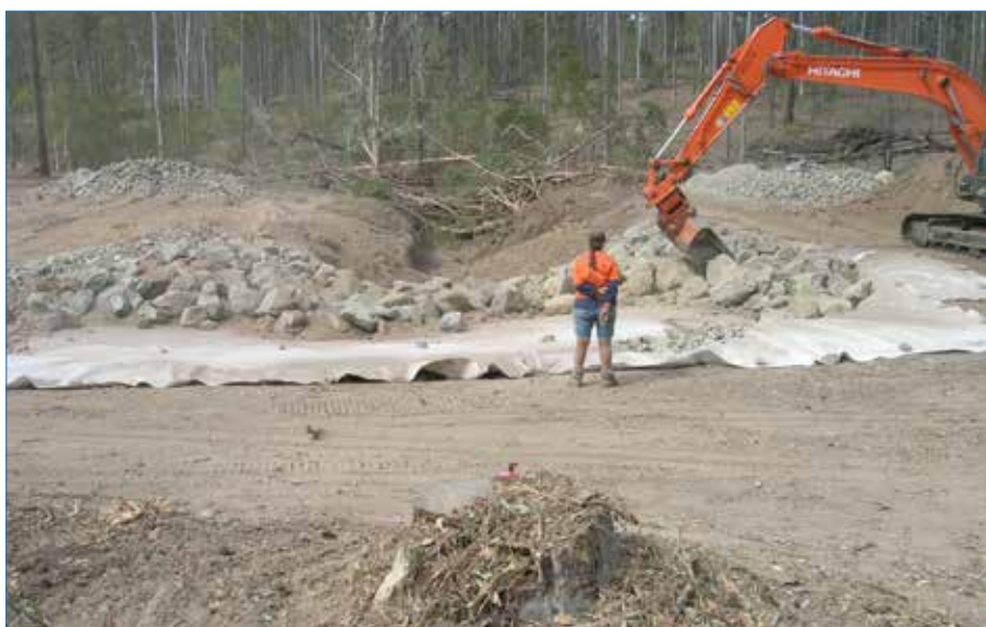
Photo 25 Geofabric laid over the chute. Rocks placed from the bottom cut-off trench to the top – due to size of chute.
