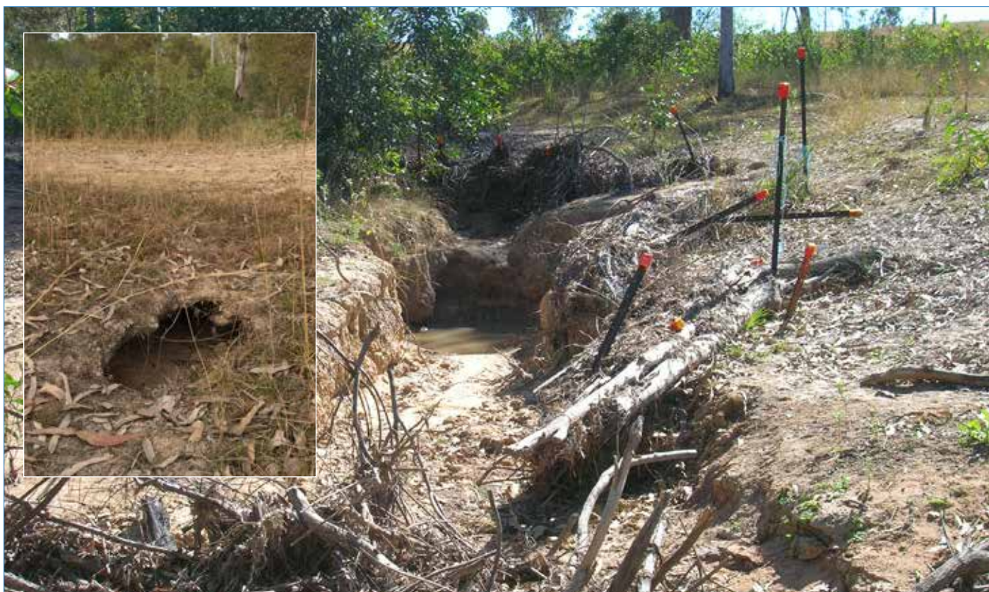
Photo 33 Gully erosion with multiple head cuts and failed porous check dams. Inset: tunnel erosion in the catchment immediately upstream of the gullies.
