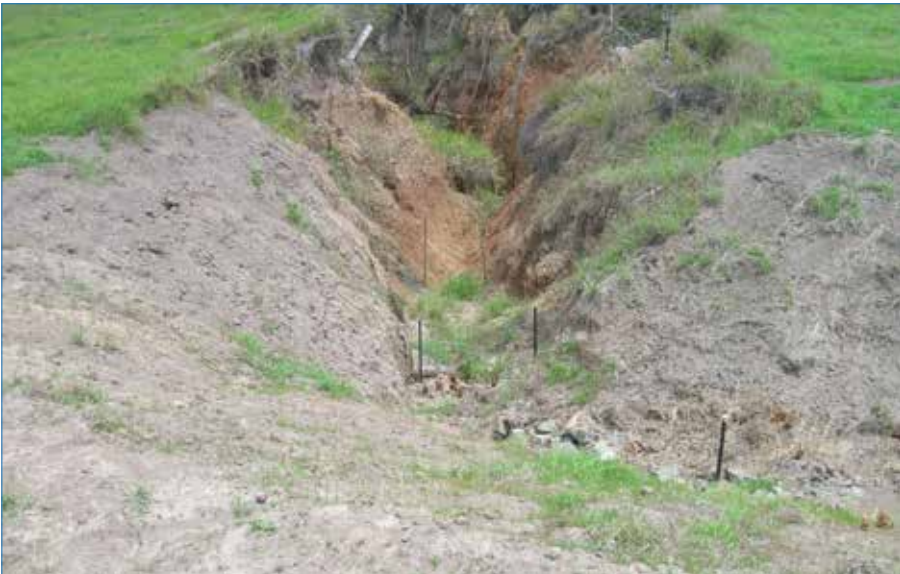
Photo 83 Gully below chute after rain, showing netting weirs.
