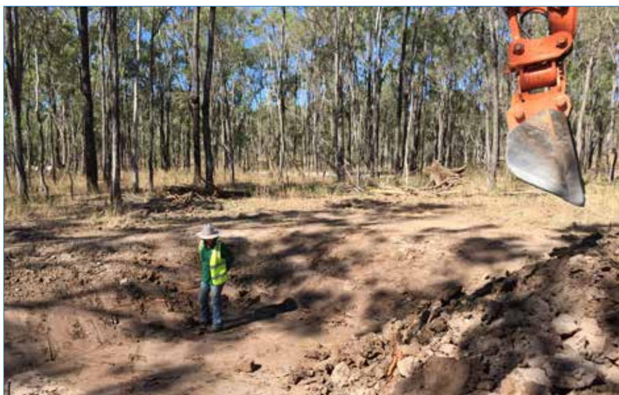
Photo 50 Detention basin taking shape.
