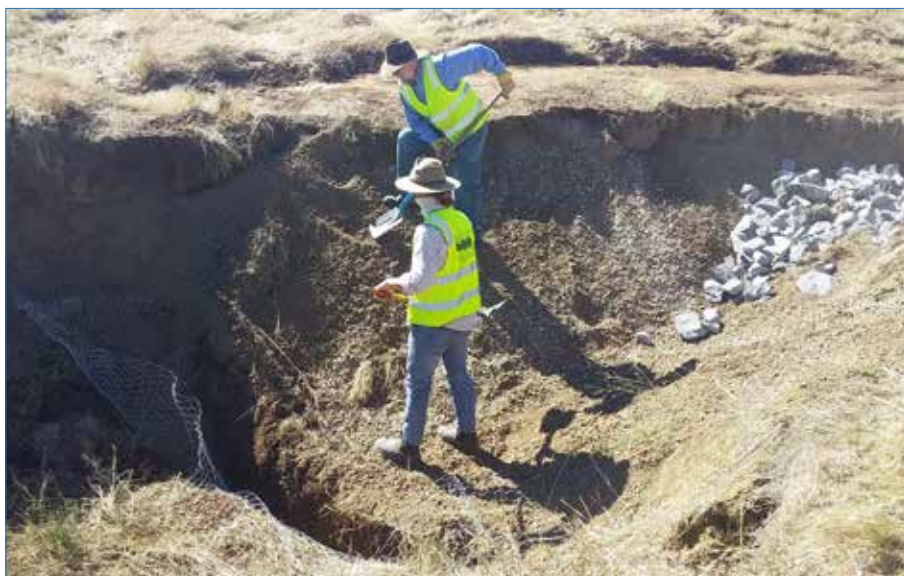
Photo 5 Bottom trench inlaid with netting and lined with clay gravel.
