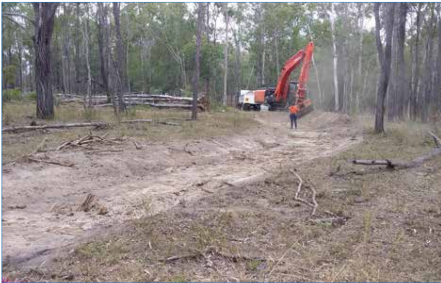
Photo 58 Levels were taken consistently along the channel floor during construction using a laser level.
