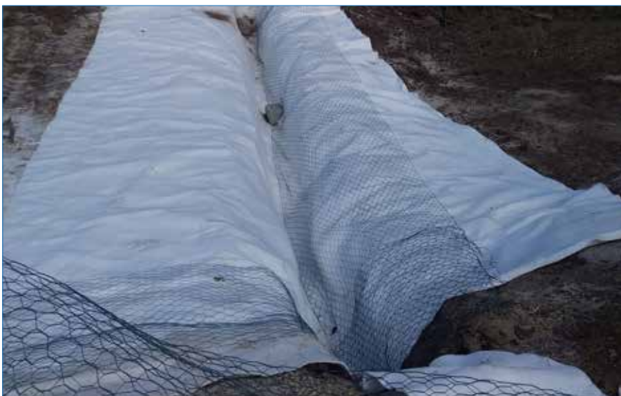
Photo 91 Completed upstream cut-off trench with geofabric and inlaid with mesh – which secured the top mesh.
