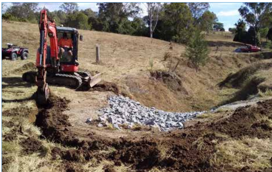
Photo 7 Excavation of top cut-off trench.
