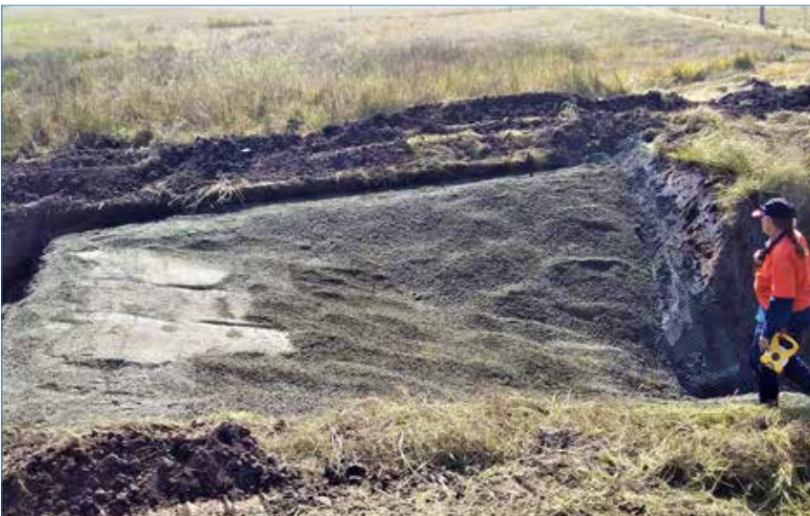
Photo 72 Chute covered with high clay gravel.
