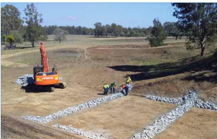
Photo 110 Rock weirs evenly spaced along the excavated site.
