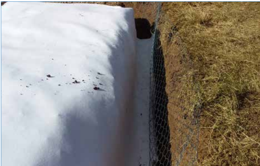
Photo 9 Geofabric Texcel R400 used to line around the full crest and over the bench only.
