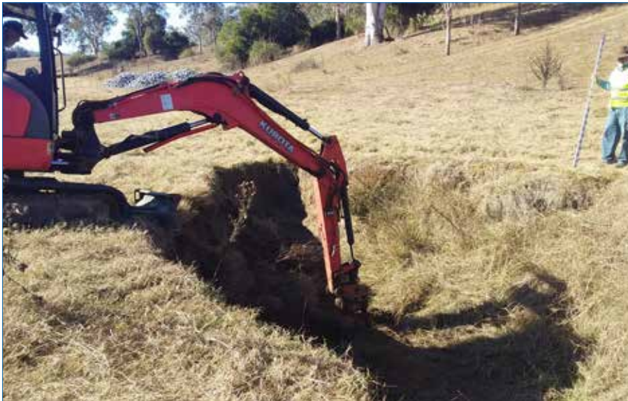
Photo 3 Dig bottom cut-off trench.
