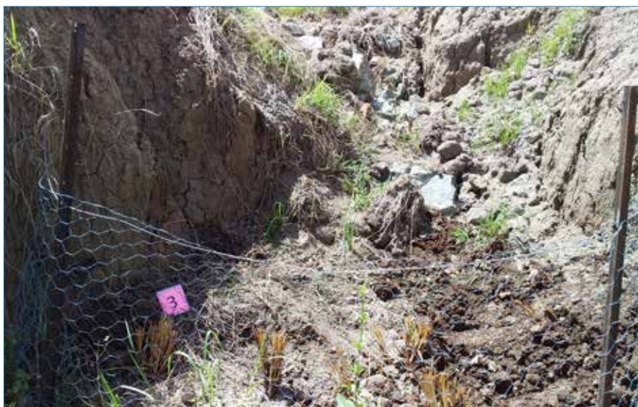
Photo 80 Construct silt trap weirs in gully floor and plant pangola grass sods.
