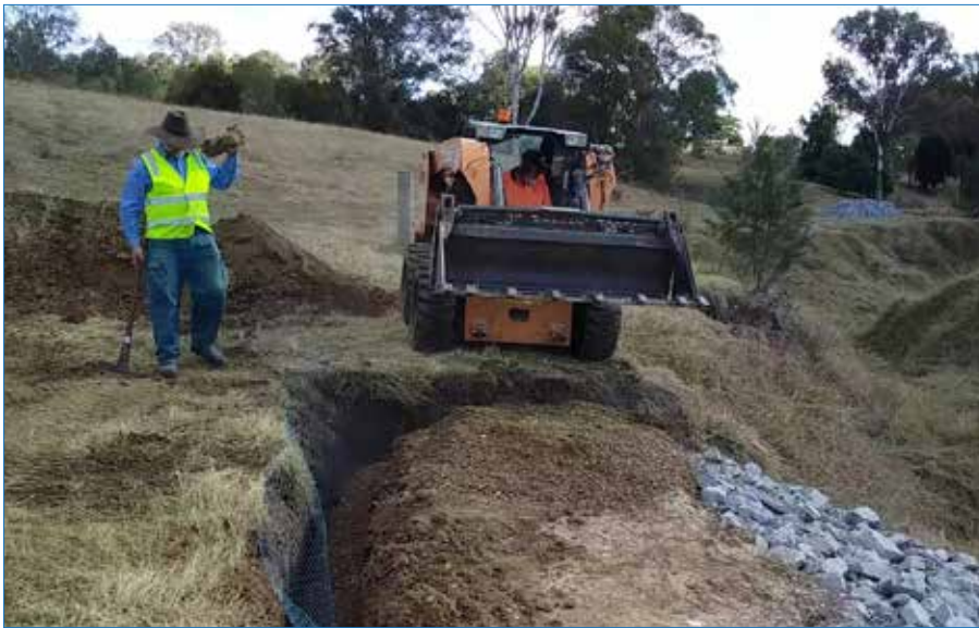
Photo 8 Wire netting and gravel placed in top cut-off trench.
