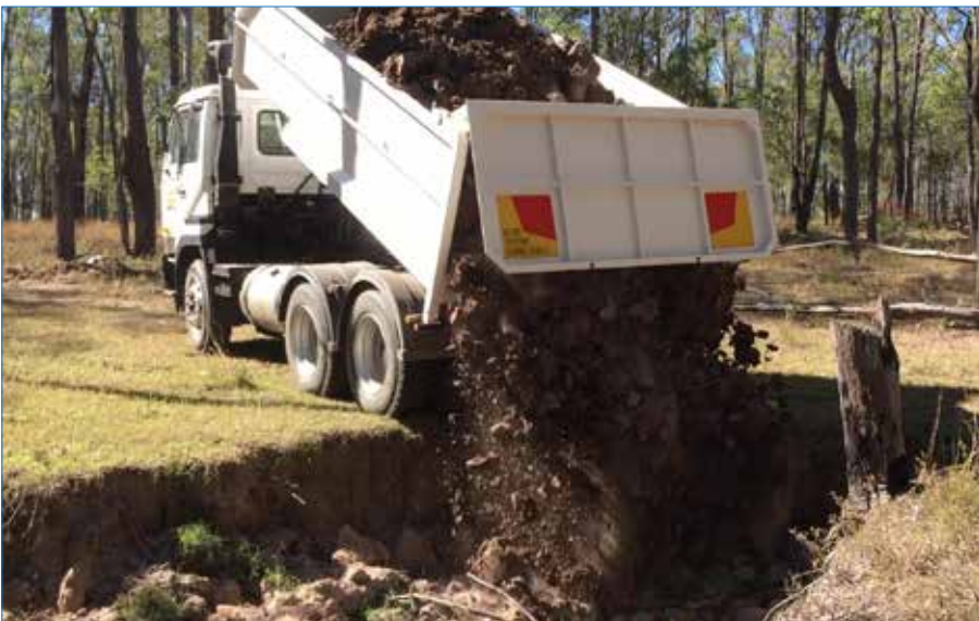
Photo 54 Spoil used to fill gully head.
