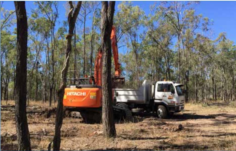
Photo 53 Excess clay soil was trucked from the detention basin site to the gully head downslope.
