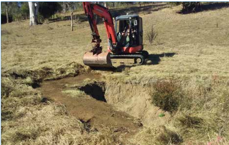
Photo 4 Prepare the crest and gully walls.
