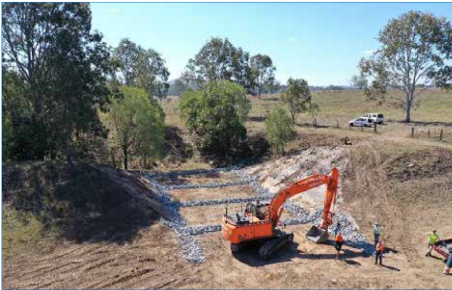
Photo 111 Completed: Looking downstream on the cut through the dam wall.
