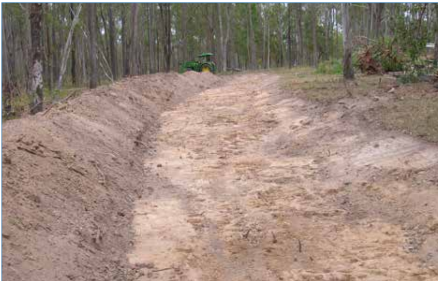
Photo 59 Completed bank looking towards level sill outlet.
