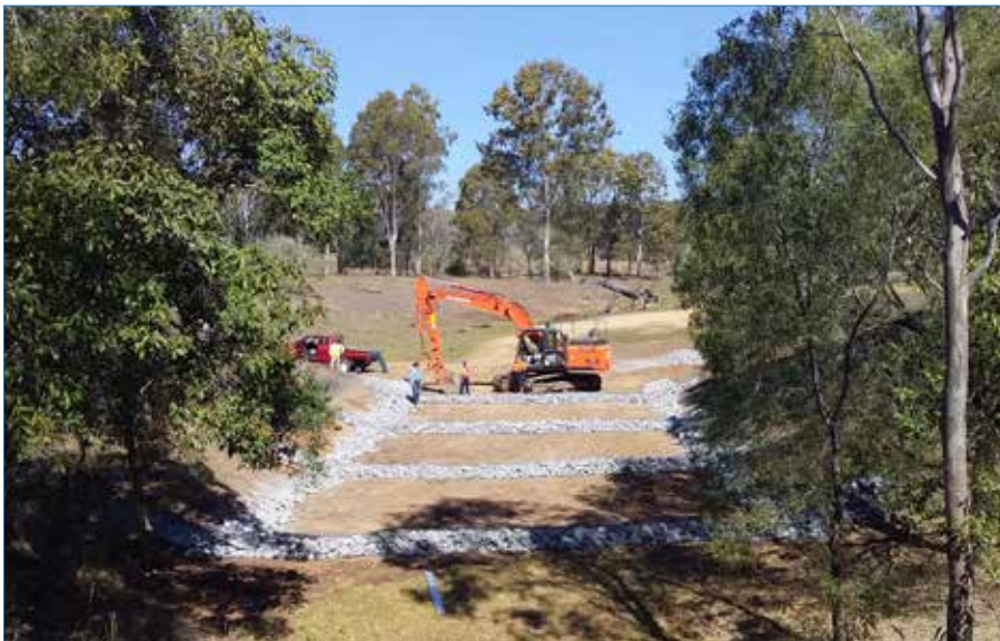
Photo 112 Completed: Looking upstream through the cut in the dam wall that reinstates the original flow path.
