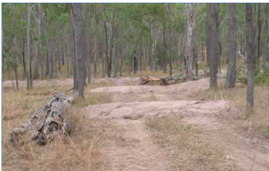
Photo 63 Whoa boys constructed on the way out to prevent erosion of tracks created during construction.
