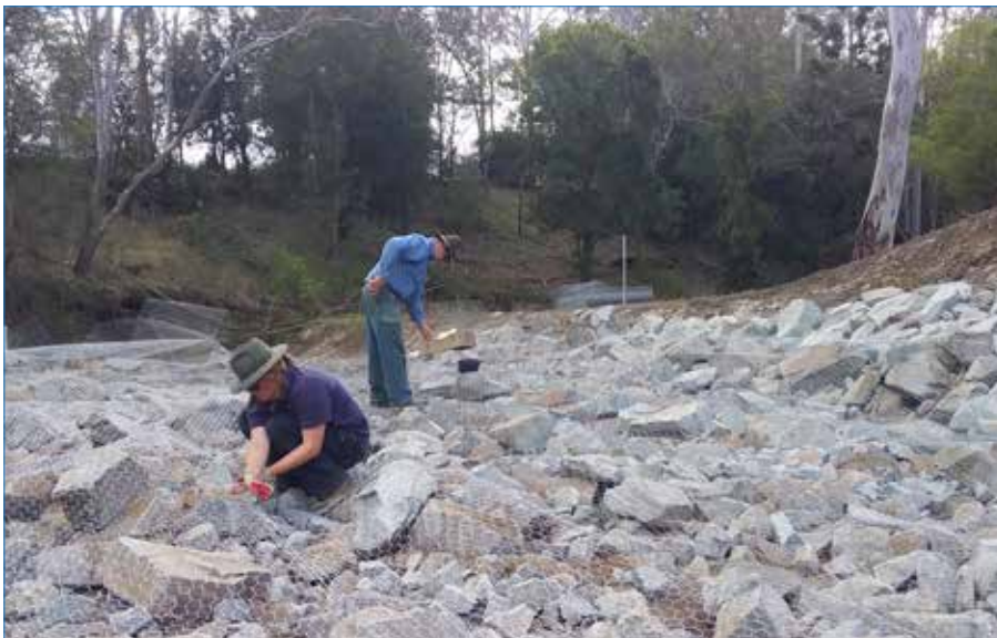
Photo 96 Covering the rock mattress with netting and stitching the overlapping lengths together starting at the upstream end.
