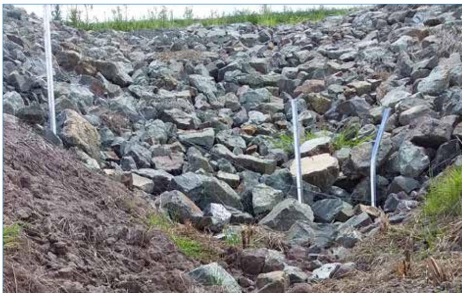
Photo 78 Place large rocks at the base of the chute for energy dissipation.
