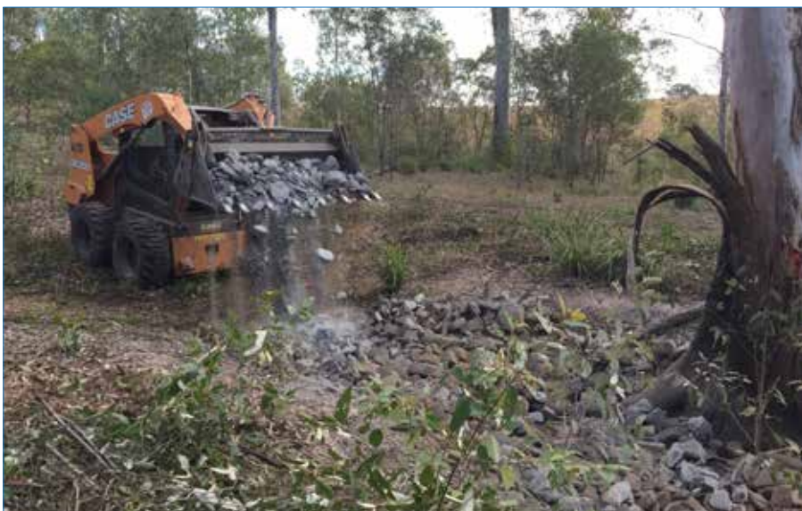
Photo 39 Fill gully head above tree.
