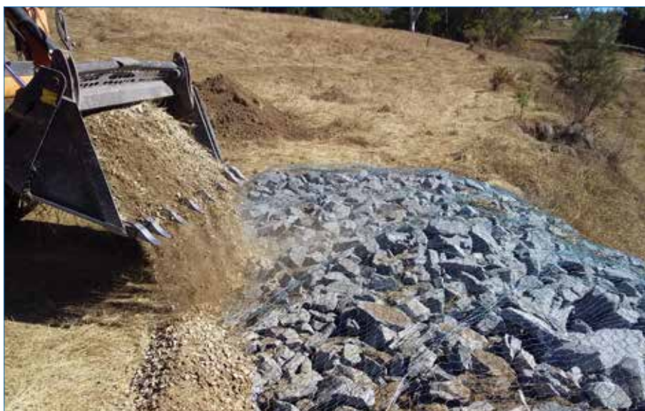
Photo 13 Filling the gaps in the rock with gravel along the crest.
