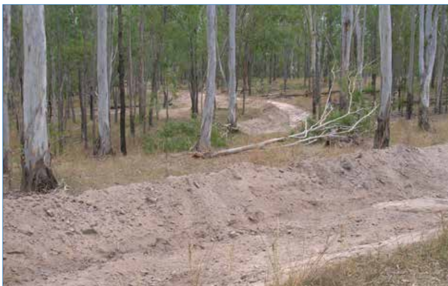
Photo 62 Background: Main diversion bank looking along the channel towards the outlet end.
