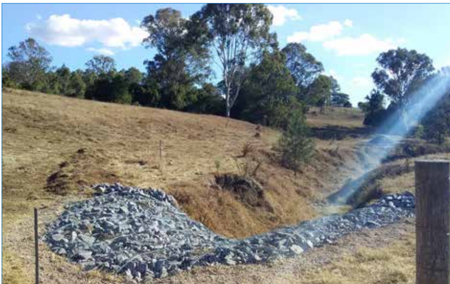
Photo 16 Looking downstream at completed chute.
