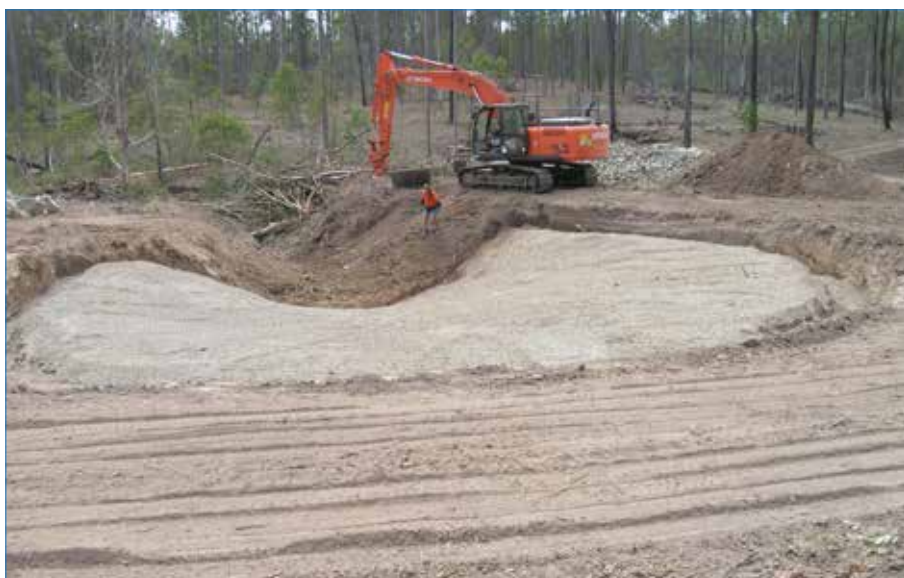
Photo 24 Cut-off trenches completed and gravel placed on batter and in trenches.
