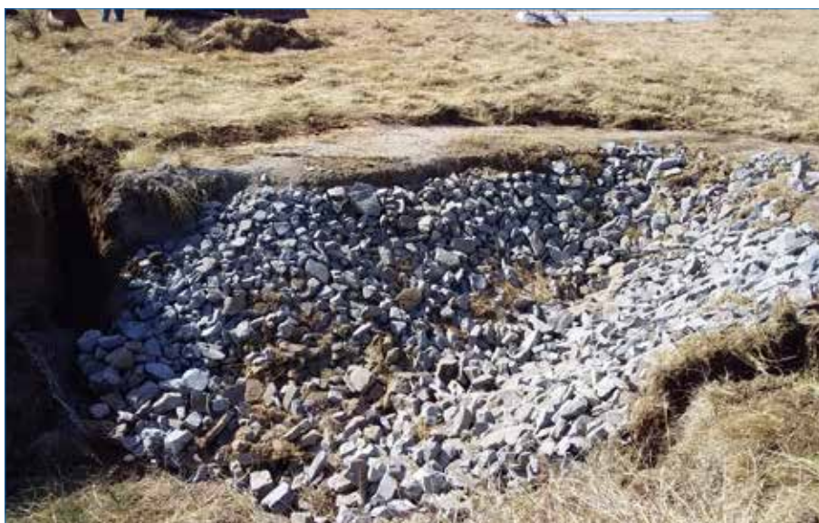
Photo 6 Trench and gully batter filled with rock.
