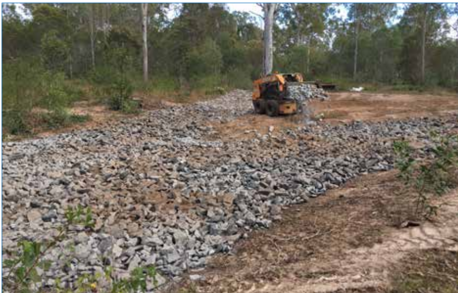
Photo 38 Finishing the rock mattress.
