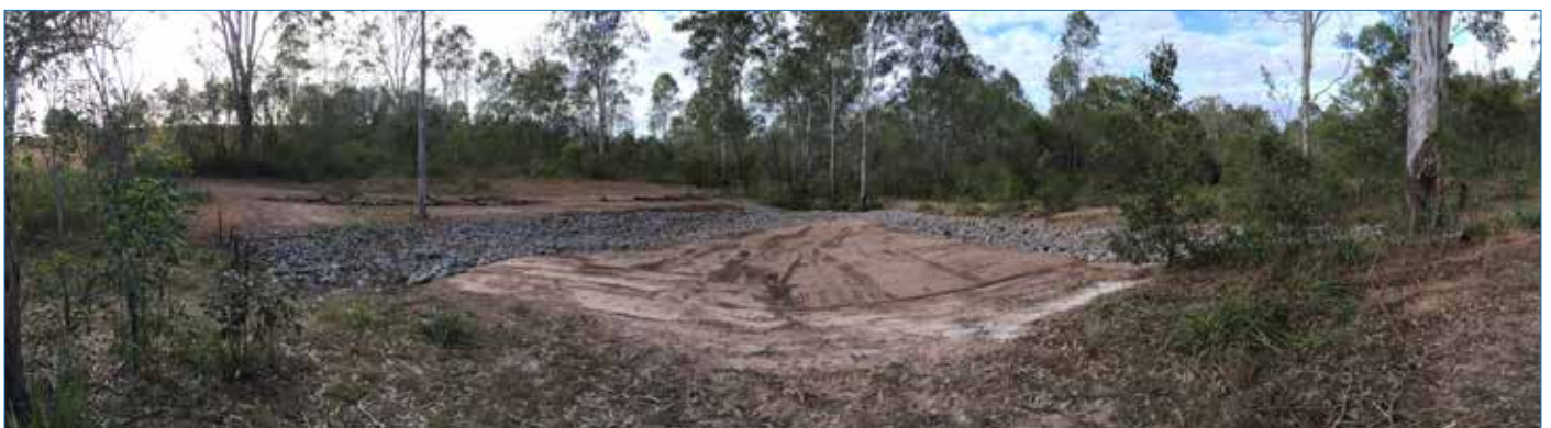
Photo 45 Looking downstream – completed project.
