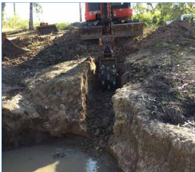
Photo 34 Exposing and compacting tunnels.
