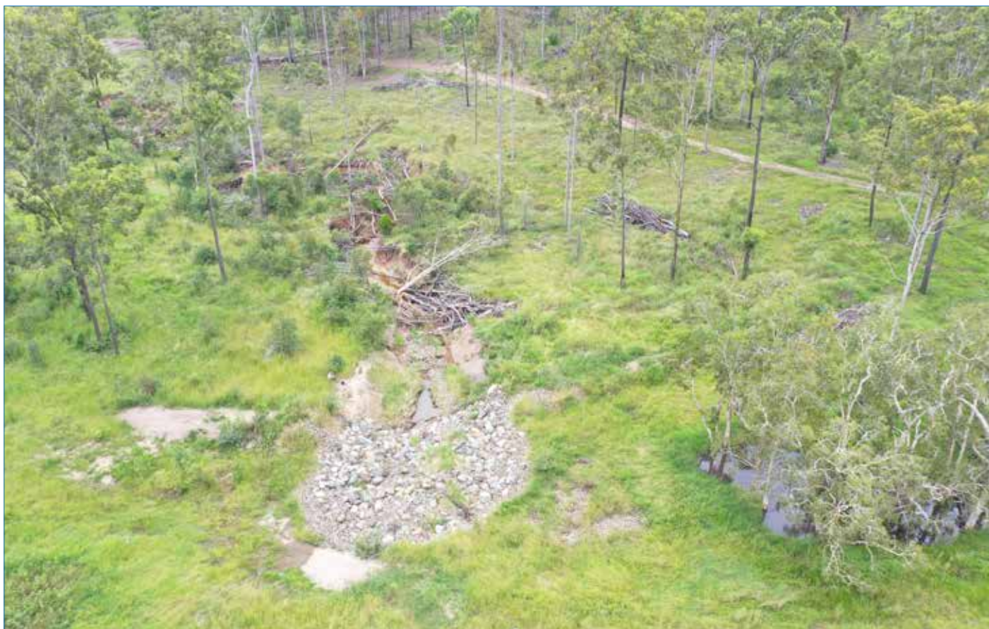
Photo 32 February 2022 after major floods in the area. 24-hour rain totals exceeded 600 mm in the area.
