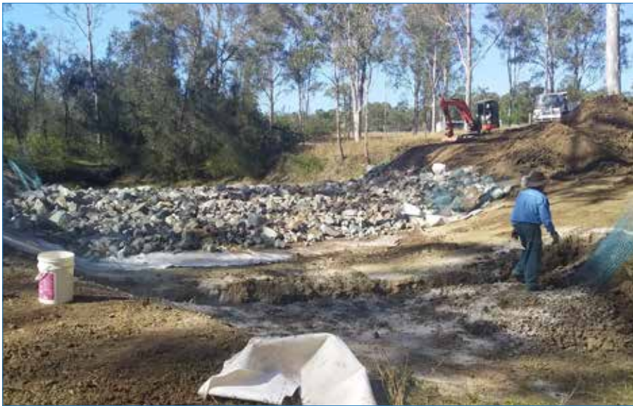
Photo 95 Looking upstream – shows the position of netting and rock mattress.
