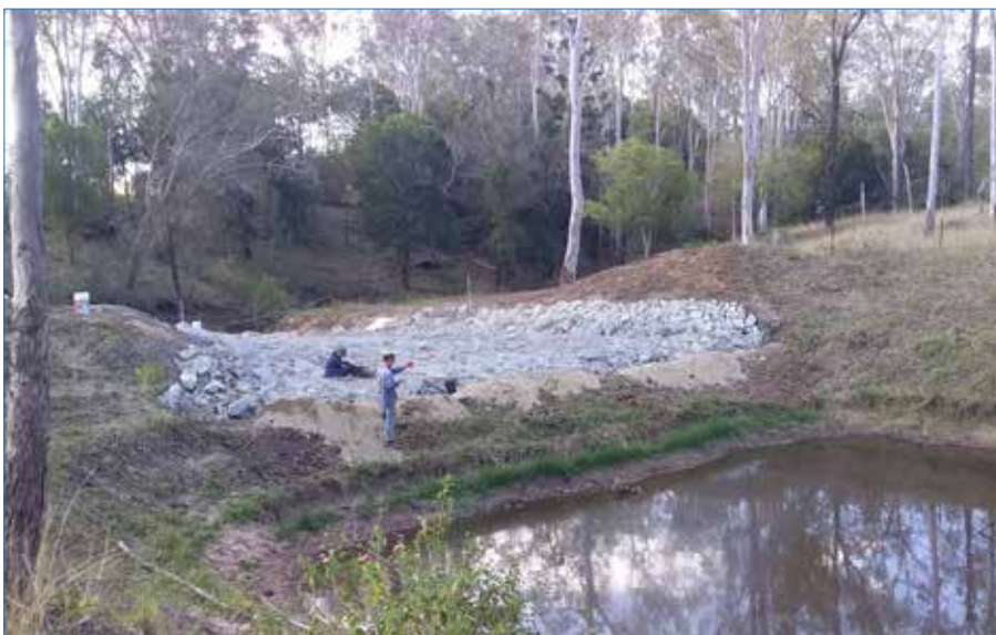
Photo 97 Gravel placed along the top cut-off trench was then shovelled by hand into the trench to fill cavities.
