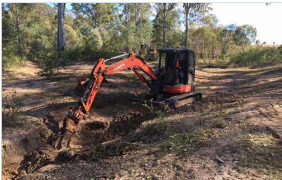
Photo 35 Filling, shaping and compacting the gully.
