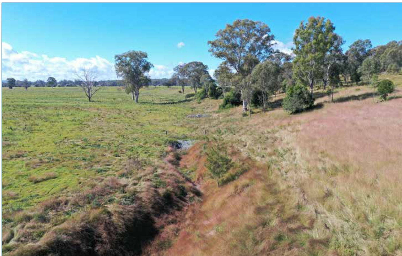
Photo 18 Ten months post-construction. May 2021 after the first wet season.
