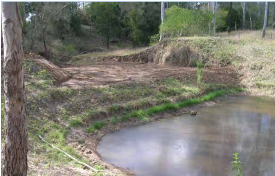
Photo 90 Dam wall cut completed to design width.
