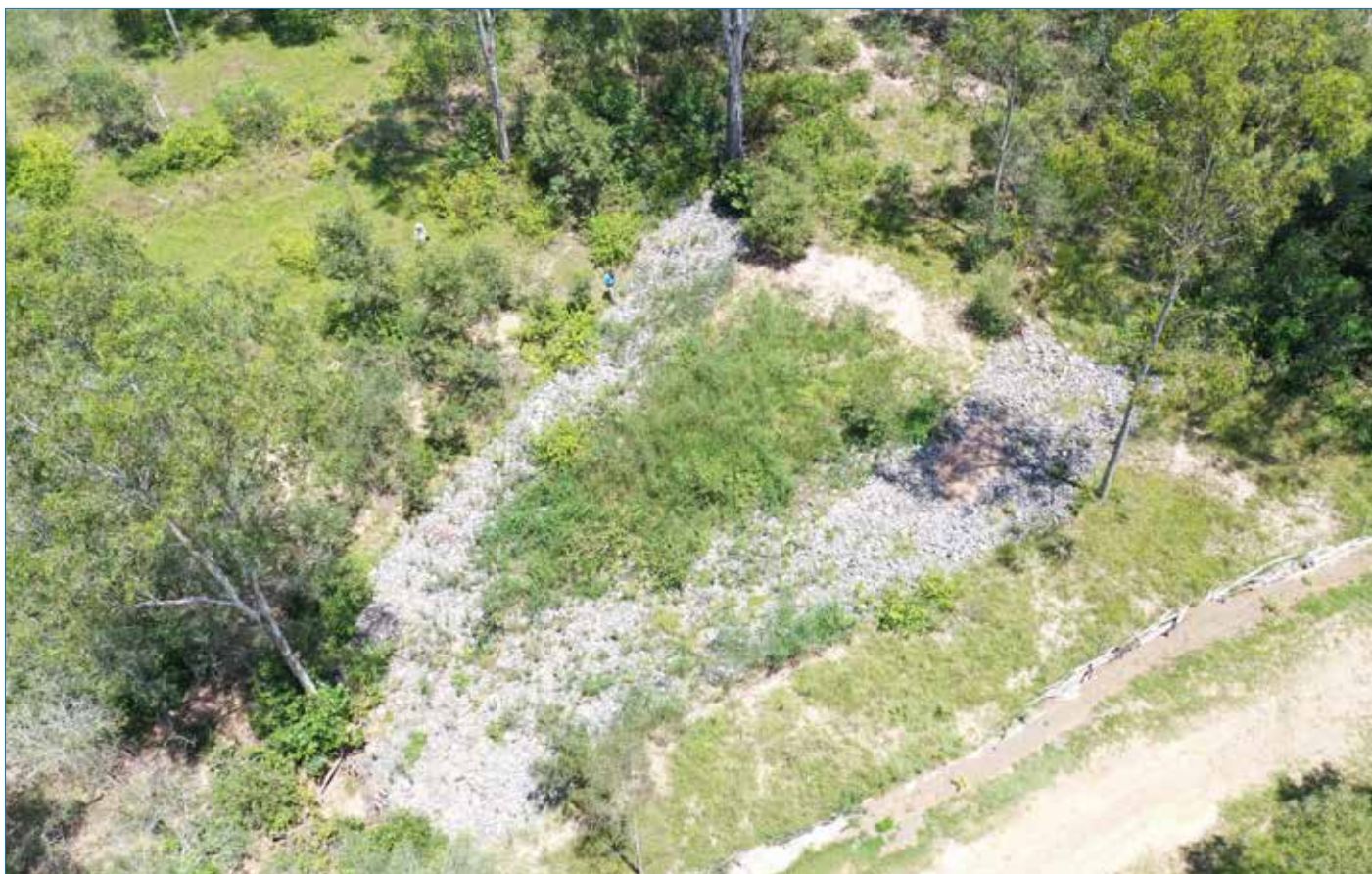
Photo 46 February 2022 after major flooding in the area.
