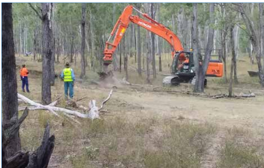
Photo 56 Clearing survey line for the main diversion bank above the gully fill.
