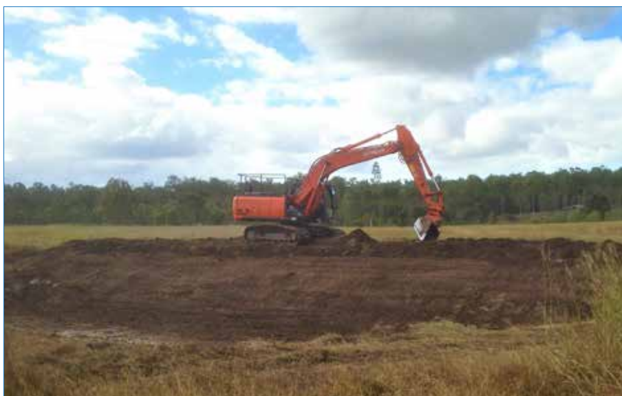
Photo 81 Detention dam construction.
