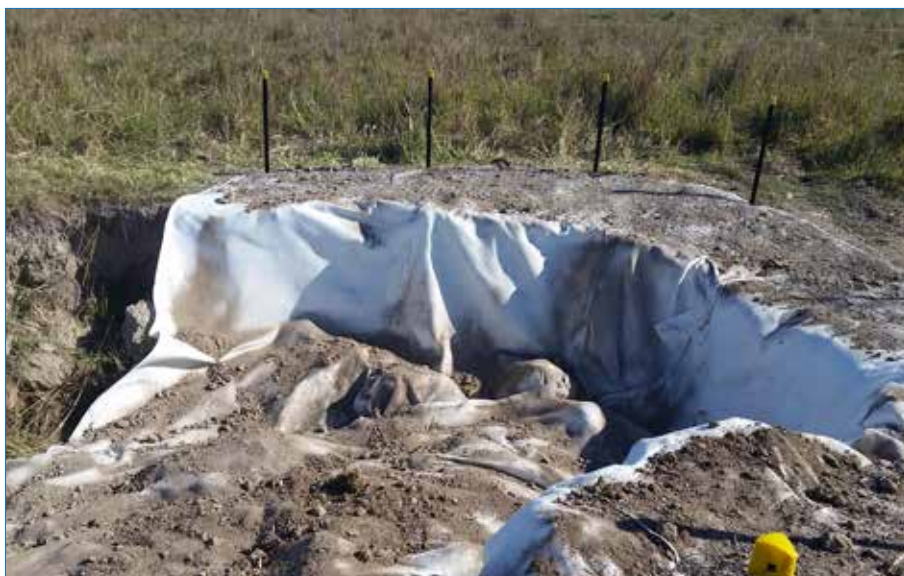
Photo 133 Mesh secured along the crest and joins stitched.
