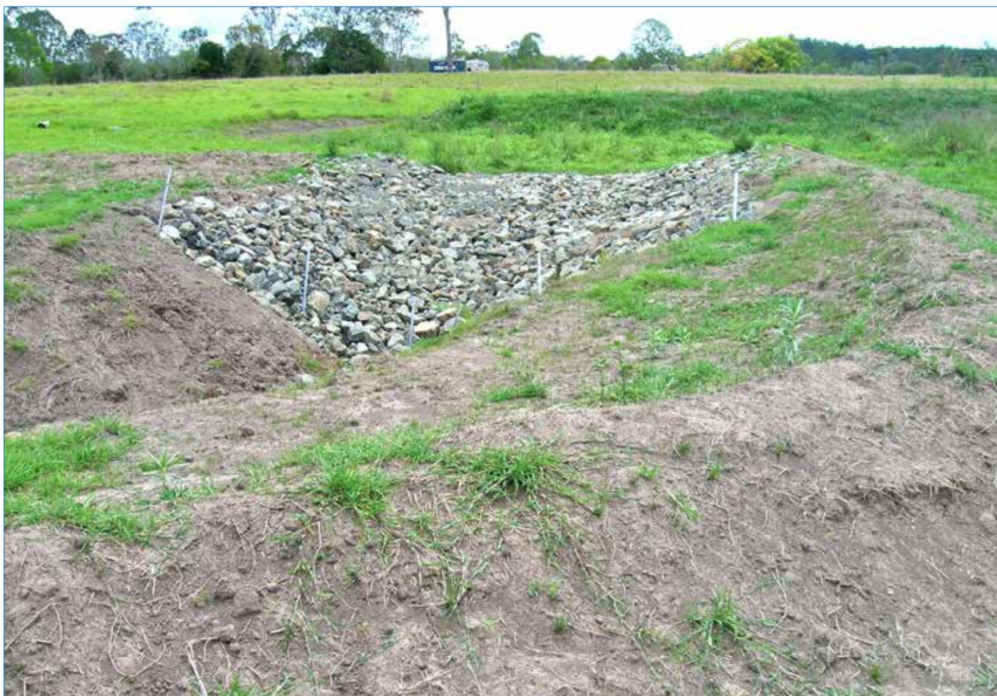
Rock chutes are an effective method to rehabilitate a wide variety of gully situations.
