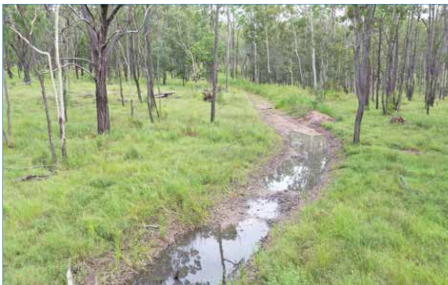
Photo 67 February 2022 post-flood. Level sill at outlet still holding some water following the flood.
