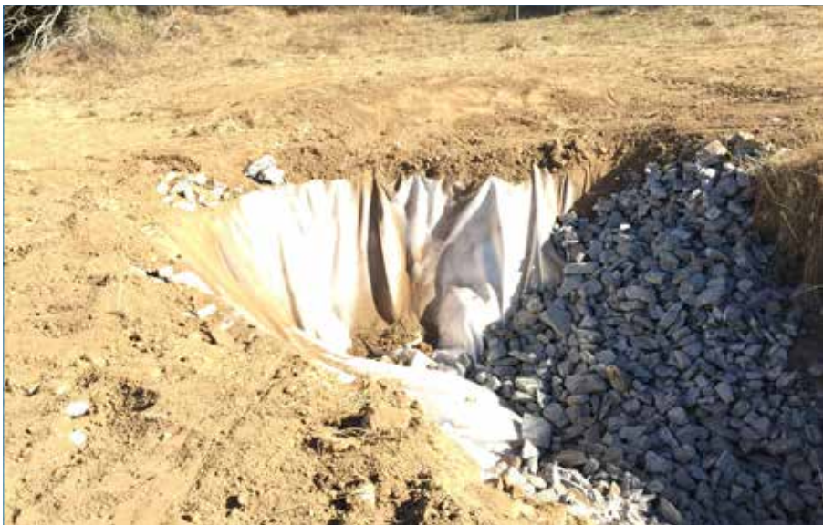
Photo 125 Covering the cut-off trench rock-fill with topsoil to encourage revegetation.
