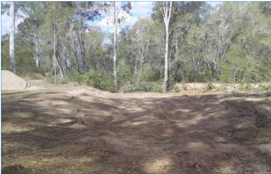
Photo 37 Gully shaped ready for gravel and rock.
