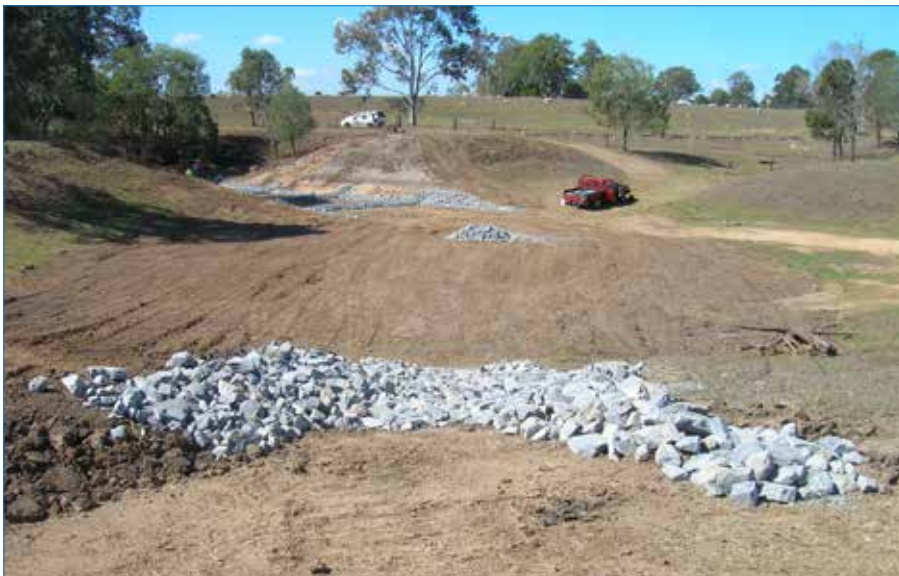
Photo 115 Completed: looking from the rock chute constructed to take the water from the flat down to the stream bed.
