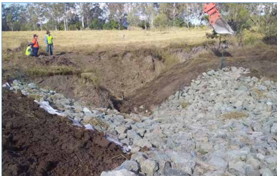
Photo 76 Batter gully walls to encourage grass growth.
