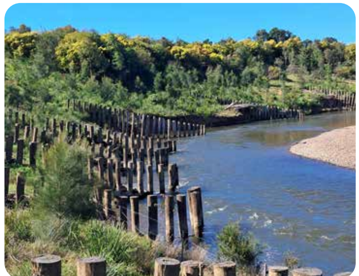
River bank repair project: before and after.
