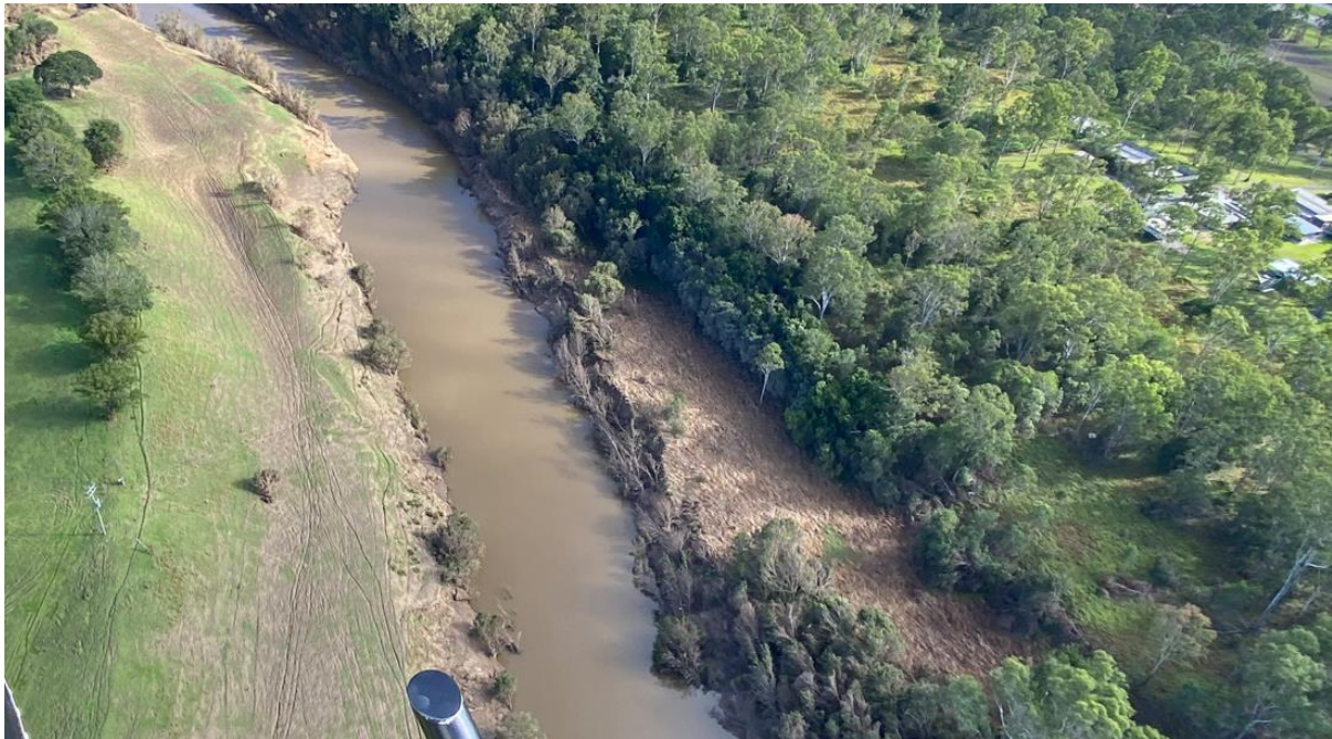
Figure 48. Example of section of bank with a moderate erosion potential in Sub-reach 3
