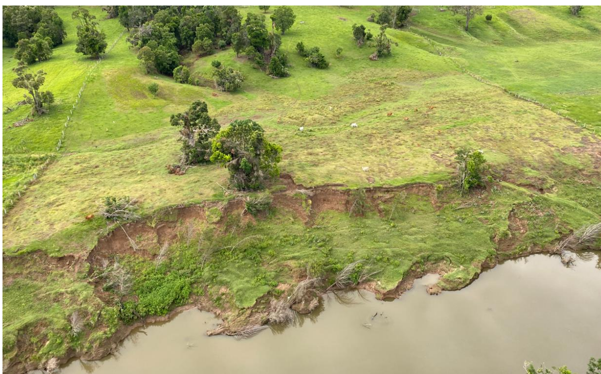
Figure 26. Example of section of bank with a moderate erosion potential in the lower portions of Sub-reach 1.
