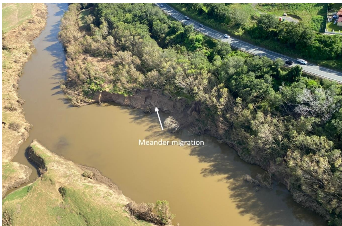
Figure 31. Active meander migration on the northern bank approximately 800 m downstream of Jones Hill Weir
